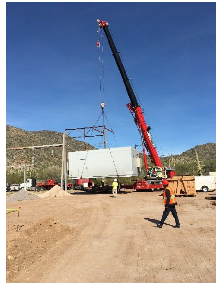
Control House Installation
